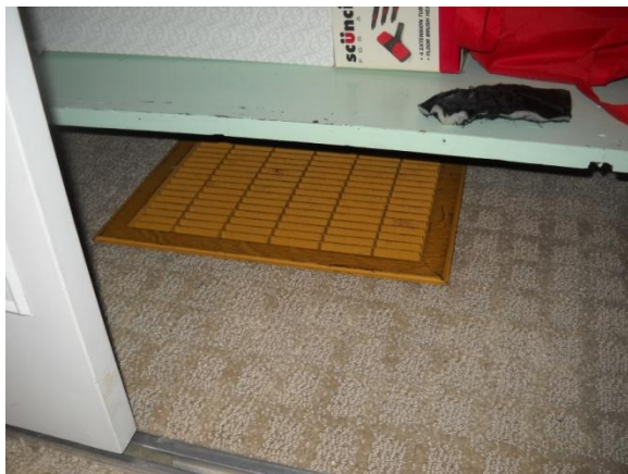
Return vents through slab at closets
