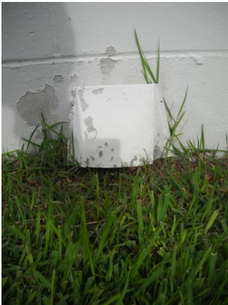
Dryer vent and condensation line terminate too close to grade (east side of home)
