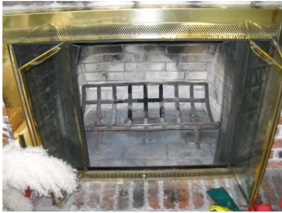
Fireplace is in good shape
