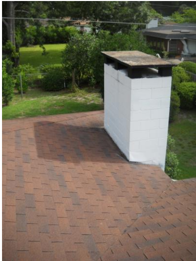
Block chimney is capped and screened
