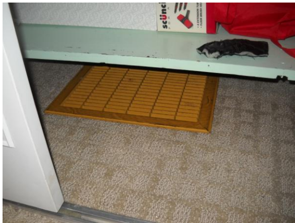
Return vents through slab at closets
