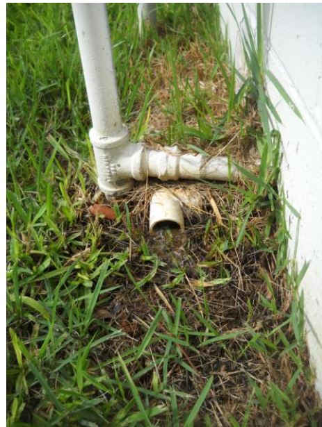
Dryer vent and condensation line terminate too close to grade (east side of home)
