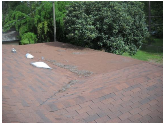
Bitumen roll roof at rear patio room
